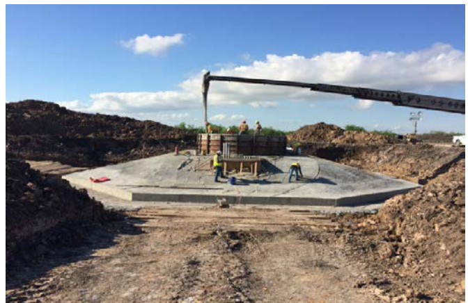
Concrete placement for turbine foundation pedestal
